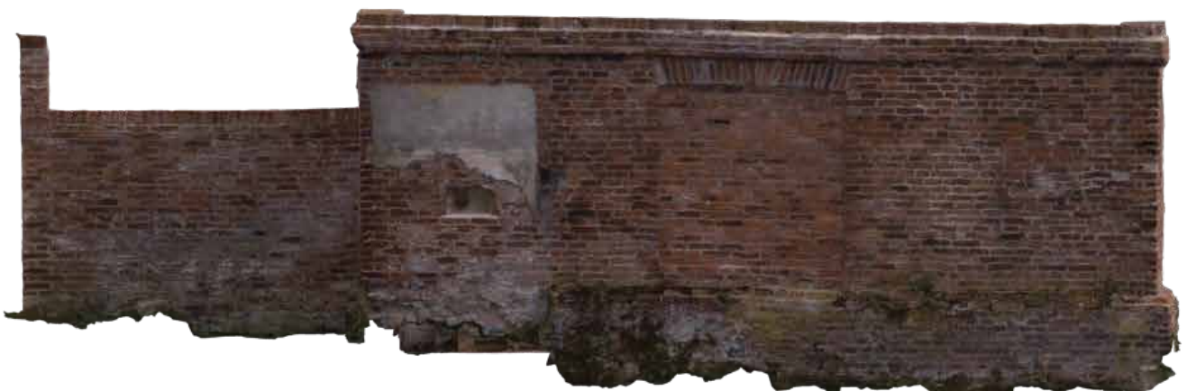
Southwest facing elevation of external wall
