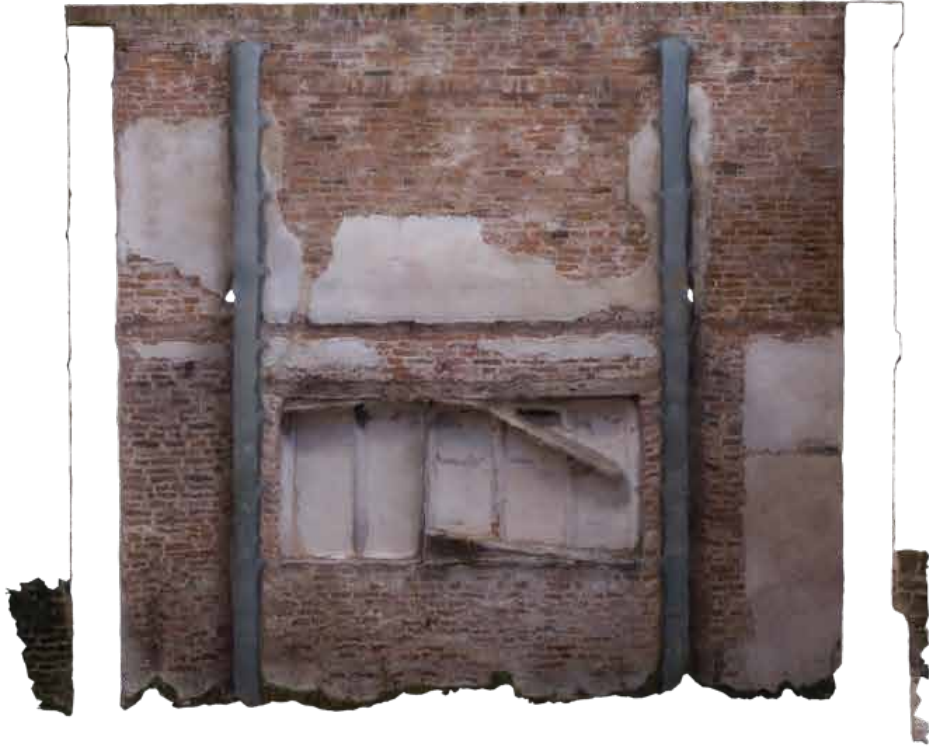
Northeast facing elevation of external wall
