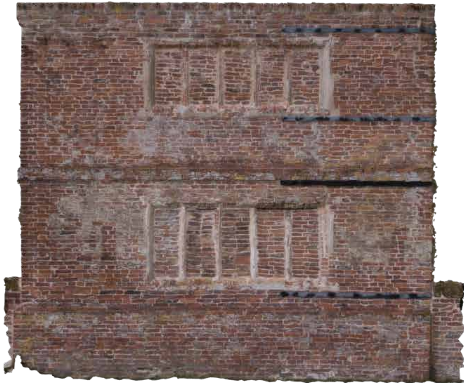
Northeast facing elevation of external wall
