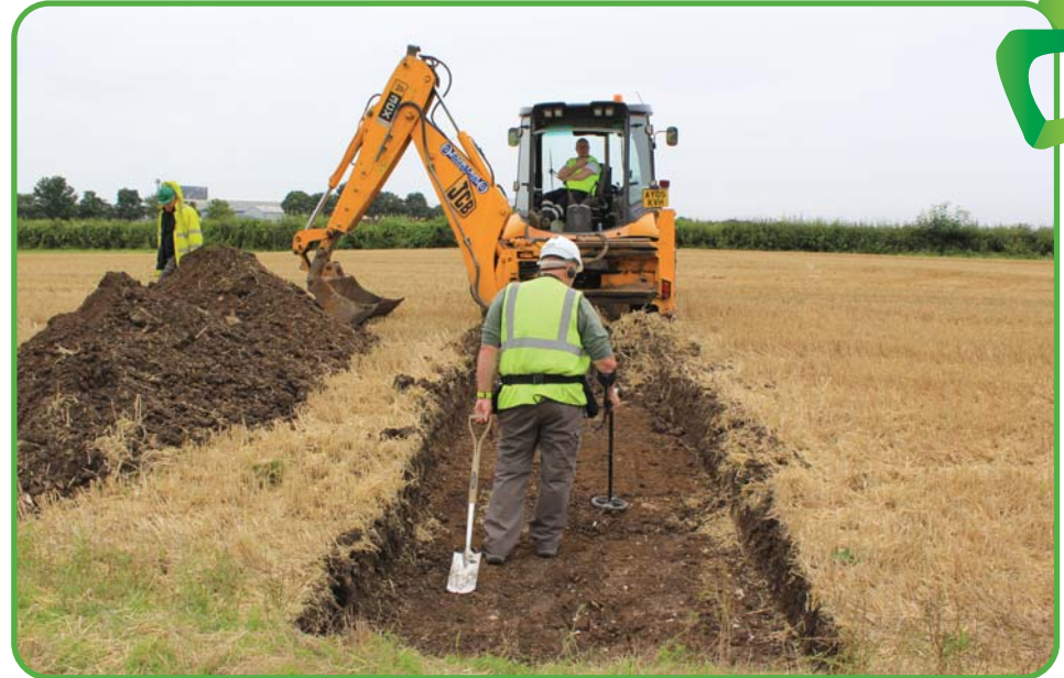
Our detectologists scanning the excavation every step of the way
